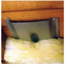
Add insulation around the rafter vent and out to the edge of the attic floor. Photo courtesy of Doug Anderson
