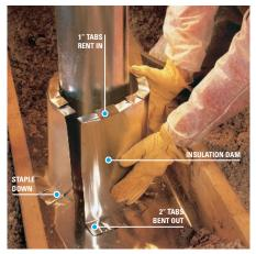
Form an insulation dam to prevent insulation from contacting the flue pipe. Cut enough aluminum from the coil to wrap around the flue plus 6 inches. Cut slots 1 inch deep and a few inches apart along the top and bend the tabs in. Cut slots about 2 inches deep along the bottom and bend out the tabs. Wrap the dam around the flue and secure the bottom by stapling through the tabs. Now put insulation back right up against the dam.
