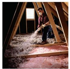
Use a blowing machine to blow in loose fill insulation. Photo courtesy of Green Fiber
