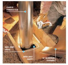
Cut aluminum flashing to fit around the flue. For round flues, cut half circles out of two pieces so they overlap about 3 inches in the middle. Press the flashing metal into a bead of high-temperature caulk and staple or nail it into place. If there's no wood, staple or nail it directly to the drywall, but be sure not to staple or nail through the drywall.
