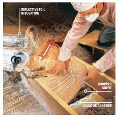
After removing insulation from a dropped soffit, cut a length of reflective foil or other blocking material (rigid foam board works well) a few inches longer than the opening to be covered. Apply a bead of caulk or adhesive around the opening. Seal the foil to the frame with the caulk/adhesive and staple or nail it in place, if needed.
