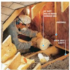
Cut a 24 inch long piece from a batt of fiberglass insulation and place it at the bottom of a 13-gallon plastic garbage bag. Fold the bag over and stuff it into the open joist spaces under the wall (a piece of rigid foam board sealed with spray foam also works well for covering open joist cavities). Again, cover with insulation when you're done.
