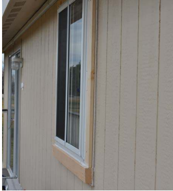
Figure 3.2. Mounting Surface for Exterior Storm Windows in Lab Homes B
